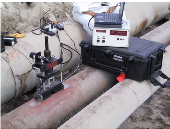
Fig. 1 Photographs of the 14-inch diameter Kerosene pipeline in Alexandria, Egypt.
