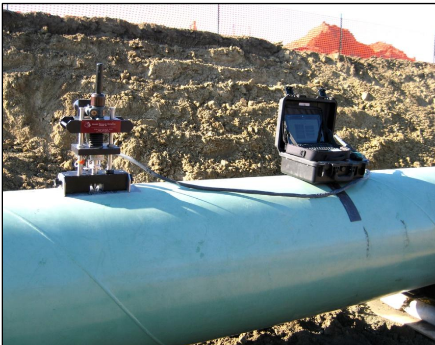
Fig. 1b In-Situ SSM system being used to test base metal of a new construction oil pipeline in order to verify the Grade of the pipeline and its actual yield strength (YS).
